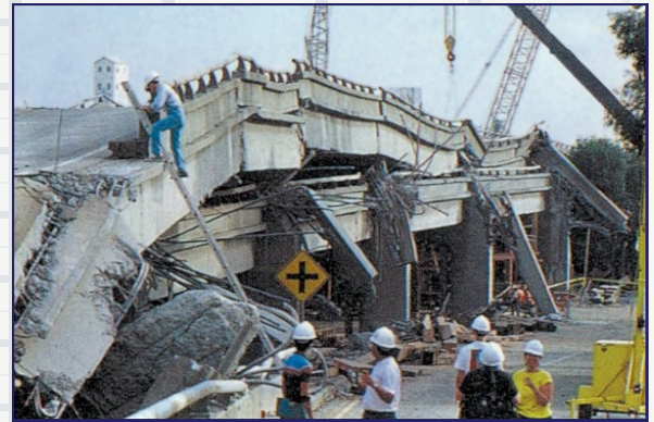
Loma Prieta, CA 10/17/1989
